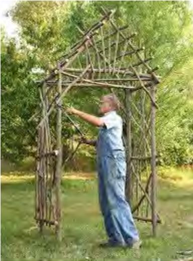
Stand the arbor upright. Add 18-inch-long sticks for corner braces to the front and back, making sure the sides are parallel. Check for any nail tips that might be sticking out and cut or bend them.
